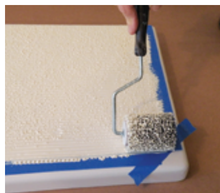
The special roller works the paint onto the surface and gives it its "grippy" texture.
